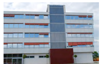
Tehnopolis building, Celje, Slovenia.
